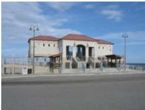
CTA Beach Comfort Station at Courthouse Rd.
