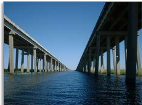
I-10 Pascagoula River Bridge
