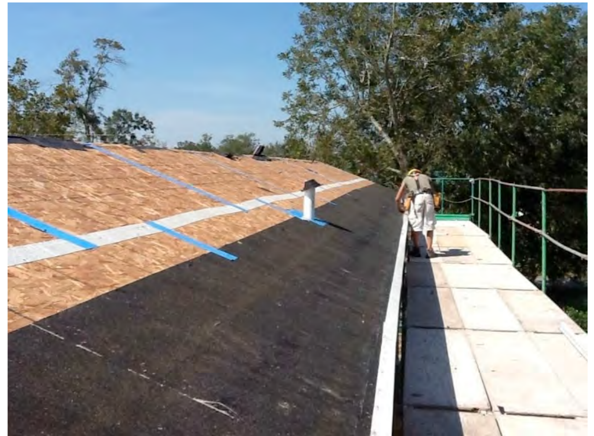
Roofing upgrades like strapping help reduce storm damage under high wind conditions.
