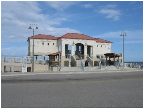
CTA Beach Comfort Station at Courthouse Rd.
