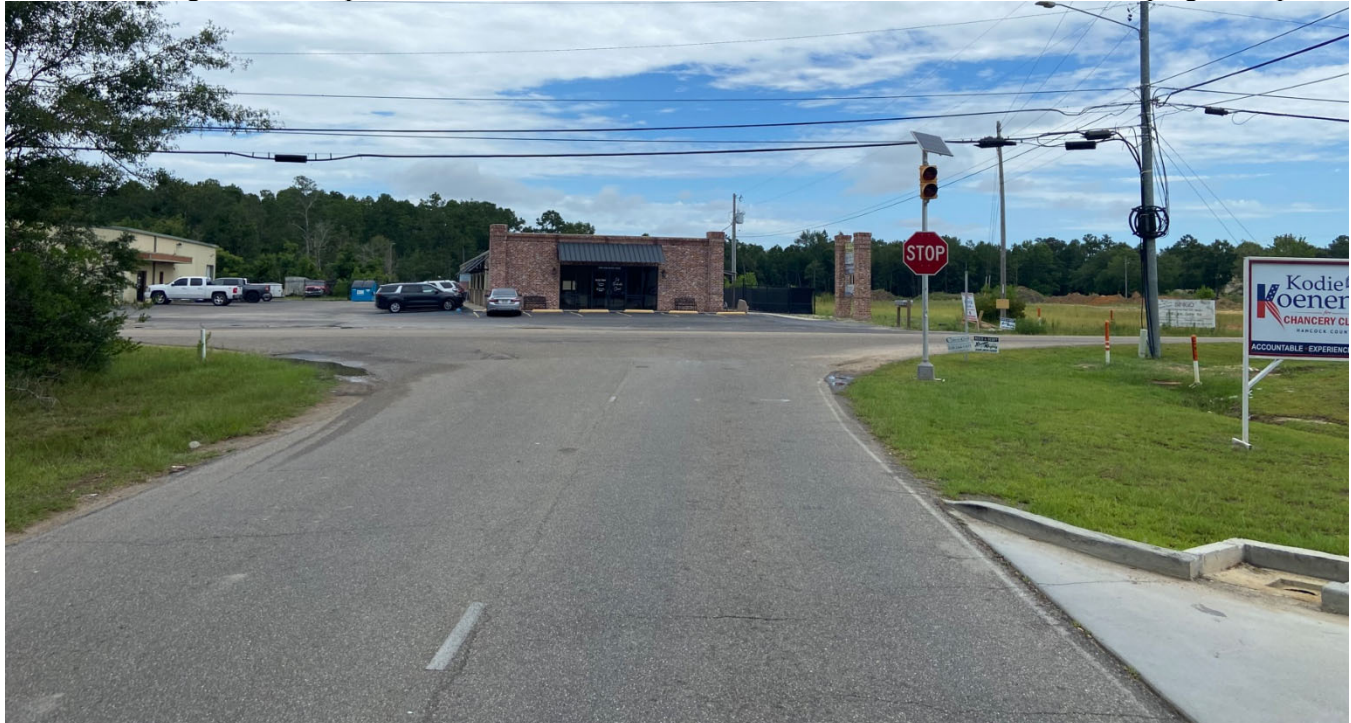
Below: Looking north on Kapalama Drive at Kiln Delisle Rd intersection and white centerline striping/no stop line.
