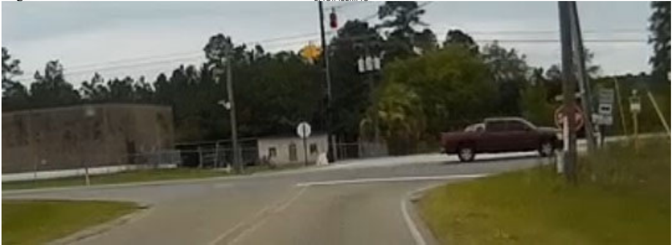
Above: Looking South on Edwin Ladner Road at Kiln Delisle Road with obscured Stop sign.
