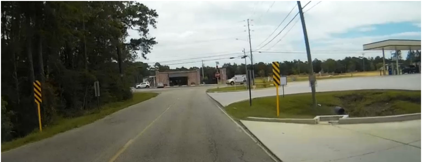
Above: Looking north on Kapalama Dr at Kiln Delisle Rd, and object markers. Marker on right is incorrect. Below: Looking south on Kapalama Drive at object makers and centerline white striping on 2-way traffic. Marker on left is incorrect.
