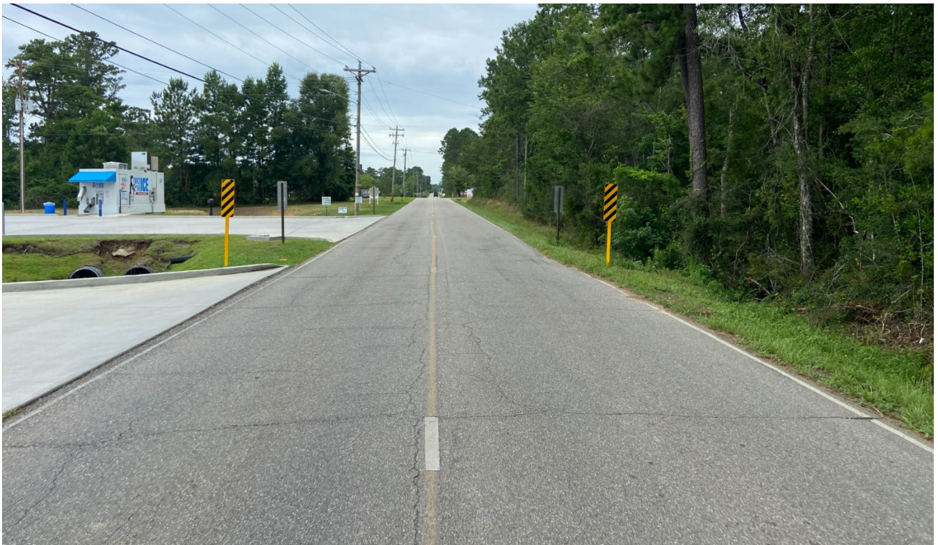
Above: Looking north on Kapalama Dr at Kiln Delisle Rd, and object markers. Marker on right is incorrect. Below: Looking south on Kapalama Drive at object makers and centerline white striping on 2-way traffic. Marker on left is incorrect.
