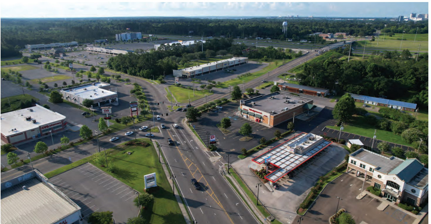
Looking south east at Sangani Blvd/Lamey Bridge Intersection
