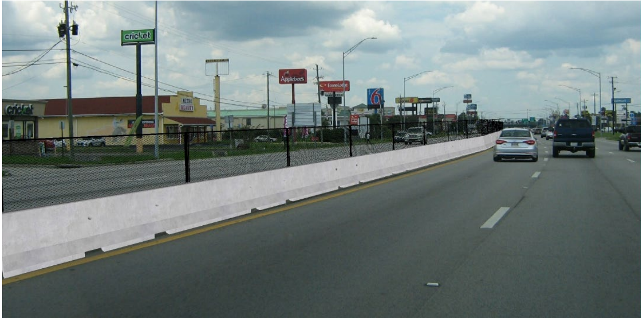
Above: 42” concrete barrier with 42” cyclone fence on top of barrier.
