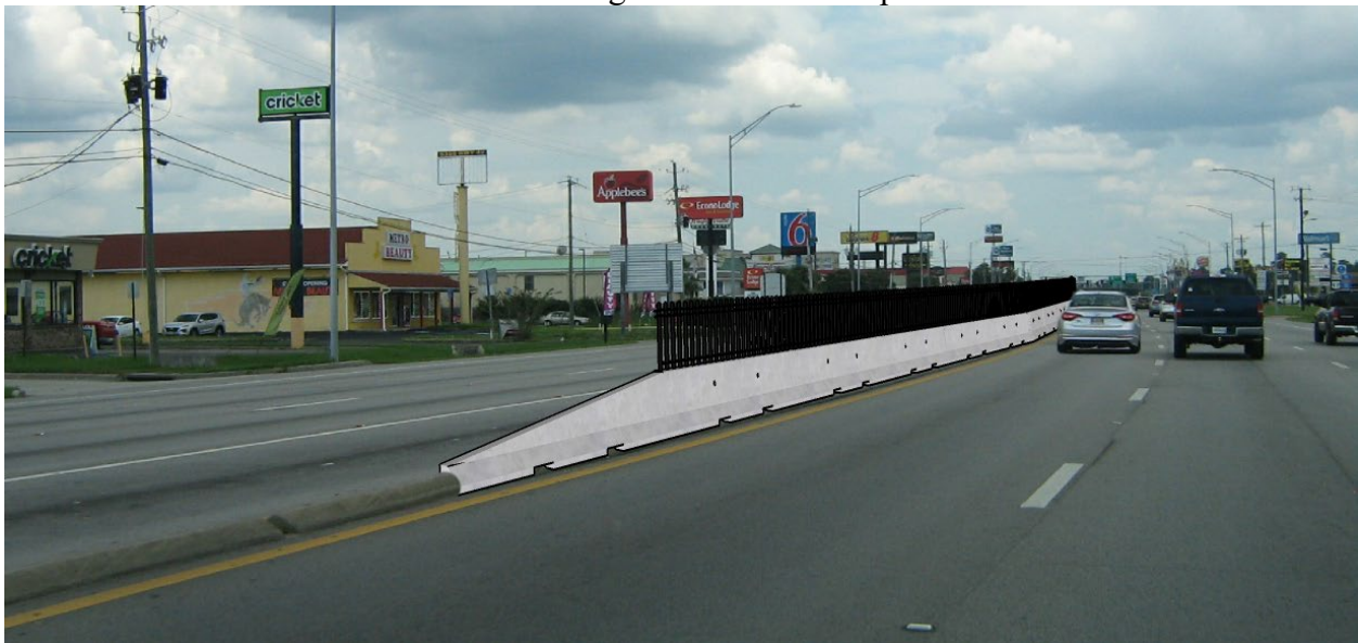
Below: 42” concrete barrier with 42” wrought iron fence on top of barrier.
