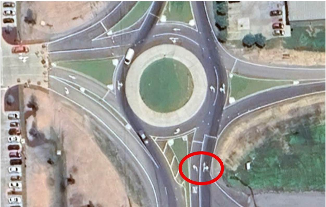
Figure 2. Northbound Roundabout Approach Improperly Marked
